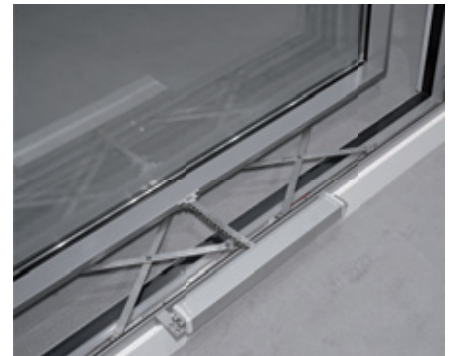
Parallel-Projecting windows Homogeneous facade design and individual ventilation
